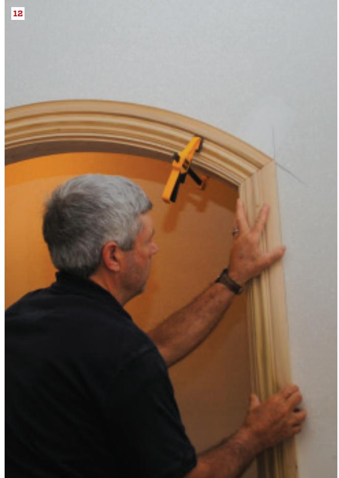
or right to find just the right place to cut the joint. With an ellipse, there is only one place to make the joint. Any small shift in position and the arch won't line up with the jamb. Most elliptical arches can be used with 8-foot ceilings.
