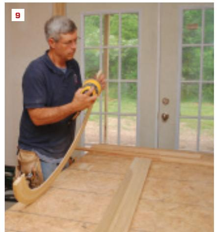
same time you make the arched molding. That way, the profile and thickness will most closely match.
